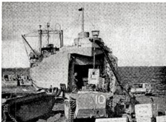
LST DELIVERS THE GOODS to an Arctic beach. This ship was one of many that raced against time to bring supplies to the DEW Line. Western Electric was prime contractor for this vital defense communications system which guards the United States from the Far North.
